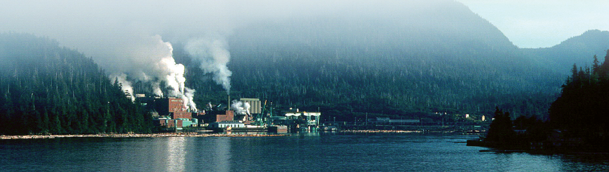
The Ketchikan Pulp Company mill in Ketchikan's Ward Cove in the early 1980s. Both the Ketchikan and Sitka pulp mills had 50-year timber contracts on the Tongass which dominated the timber industry in Southeast from the mid 1950s through early 1990s.
